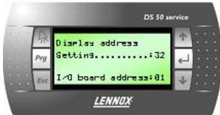
Access the configuration mode by pressing buttons ↑ ↓ ← , for at least 5 seconds until the Sds.1 screen appears:
